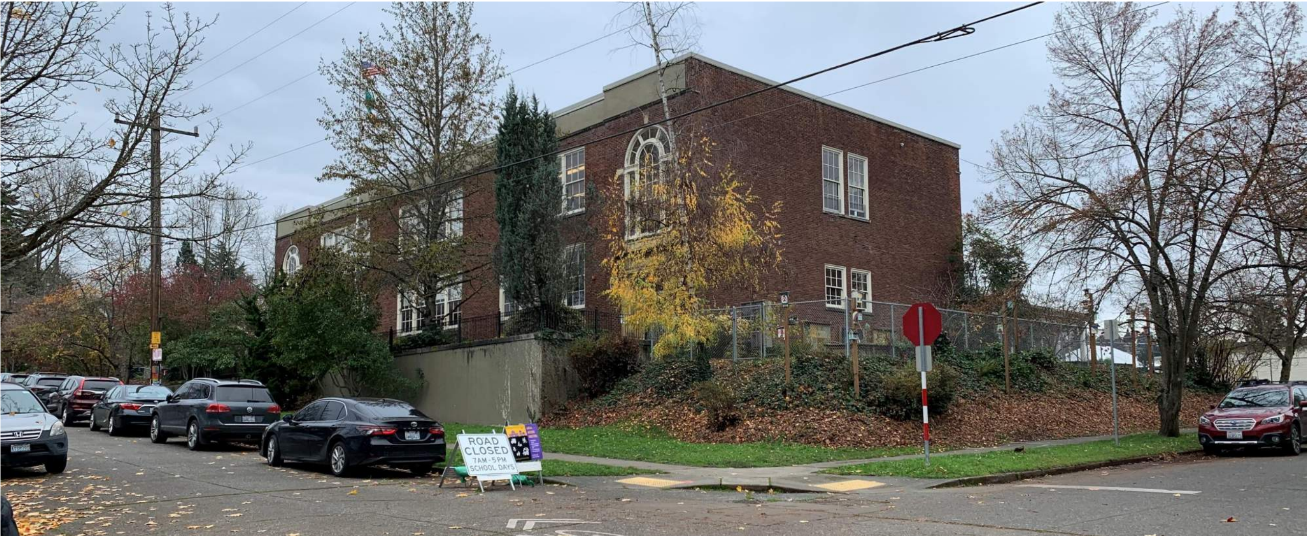
Existing Landmarked Building from corner of 22 nd Ave. E and E Calhoun St.
